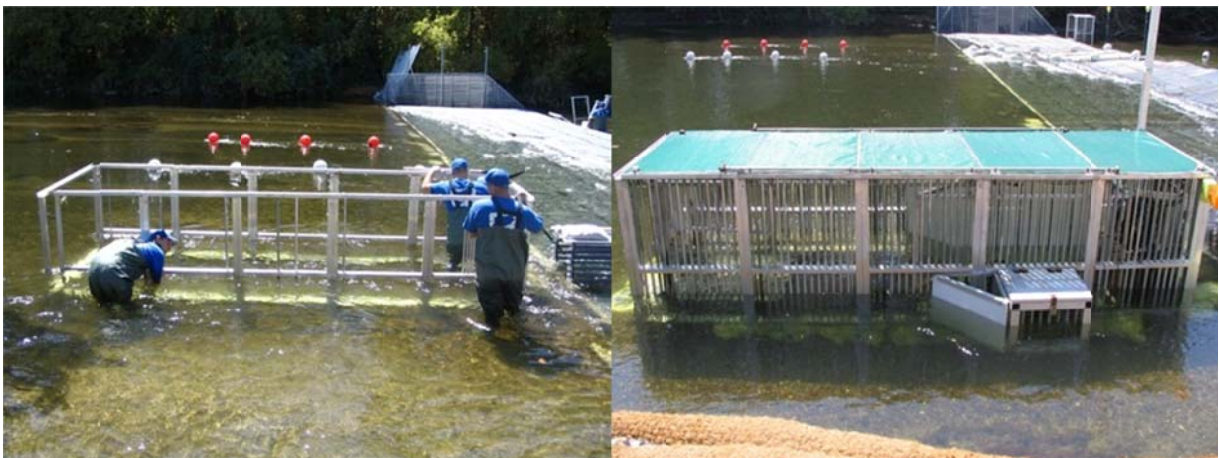
Figure 13. Initial assembly of the live trap frame (left); completed live trap installed (right).
