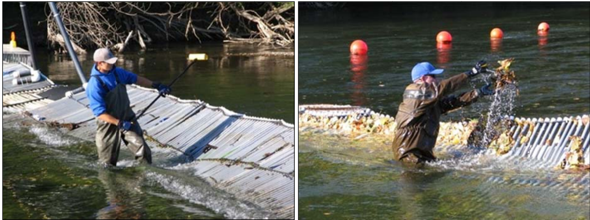
Figure 14. A technician cleaning debris from a weir using a stiff bristle brush (left); and grabbing and tossing leaf litter over the back of a weir during a high flow event (right).
