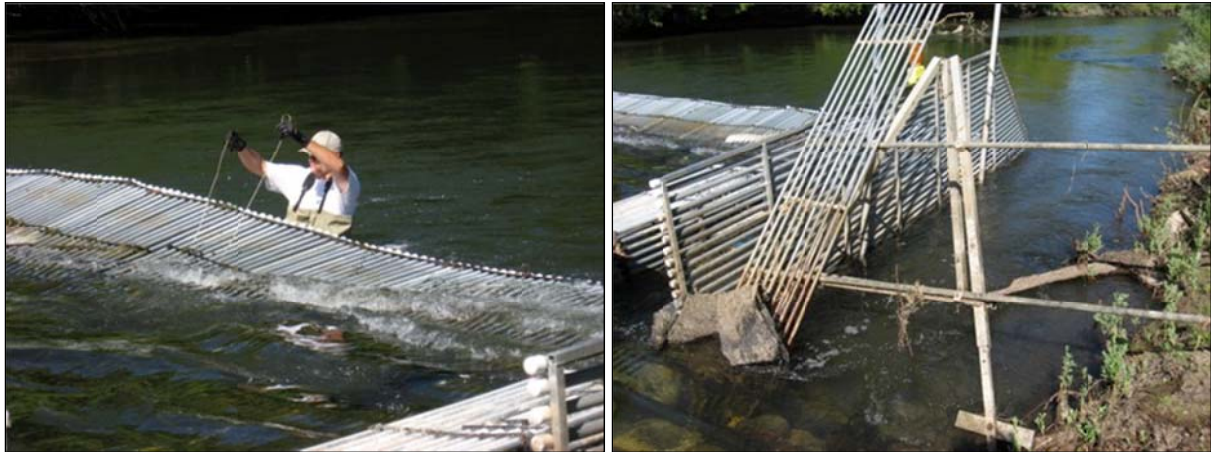
Figure 35. Technician dropping the resistance boards of an individual panel to prepare a weir for removal (left); and view of a weir with part of the rigid weir already removed (right).
